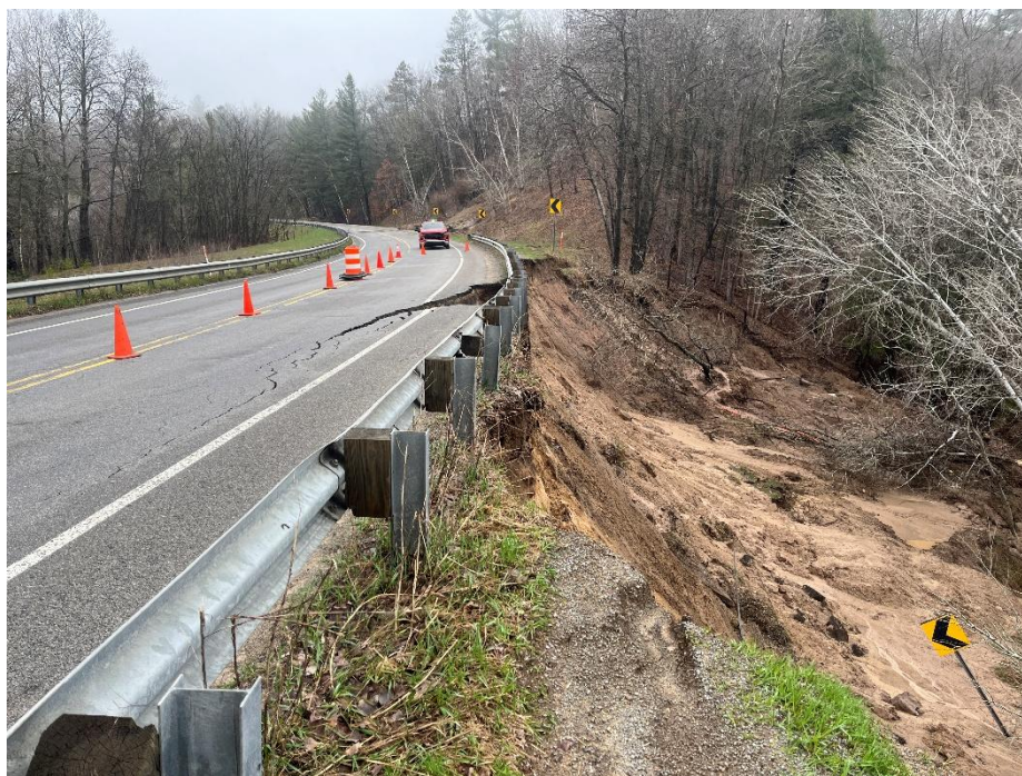
Photograph #2: View of road and southern slope adjacent to the northbound lane. (April 2026)
